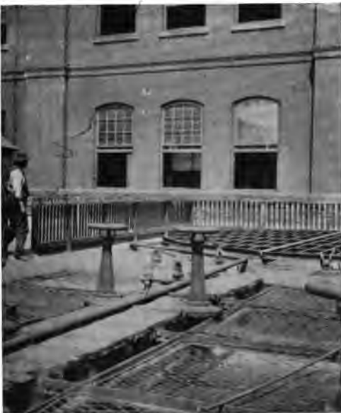
Fig. 3. Guards over Tar Separator Wells.*
